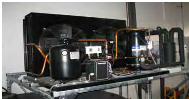
Heat recovery in the test room
